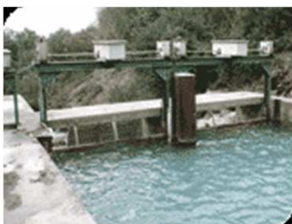
GEG hydroelectric plant
