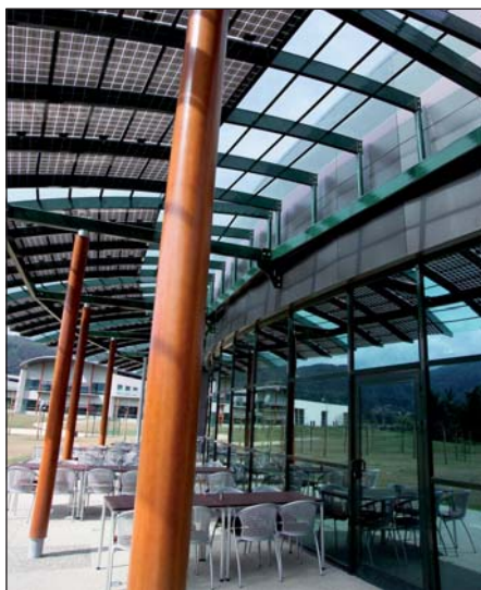
Terrace at Schneider Electric fitted with solar panels
