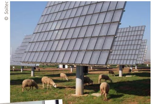
Above: a Concentrix-built concentrator photovoltaic array
